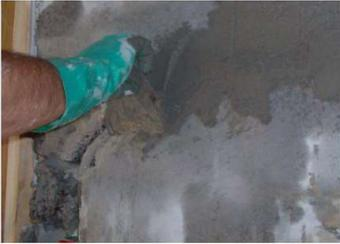
The material is based on a blend of cement, graded aggregates, special fillers and chemical additives which control the rate of set and minimise the risk of thermal cracking. Renderoc Plug provides an initial set time of approximately one minute.
