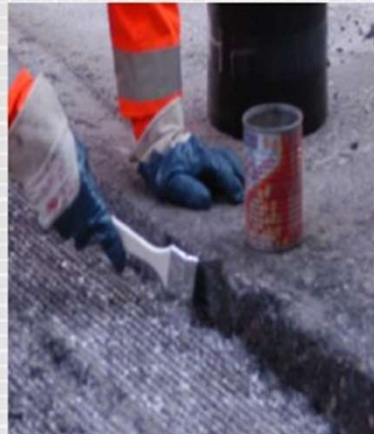
Fix-O-Flex F NV / KVV-25 / UG as joint sealing in road building
