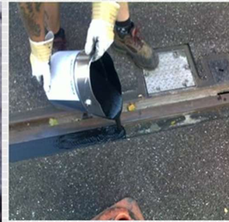
Fix-O-Flex F NV / KVV-25 / UG as joint sealing in road building
