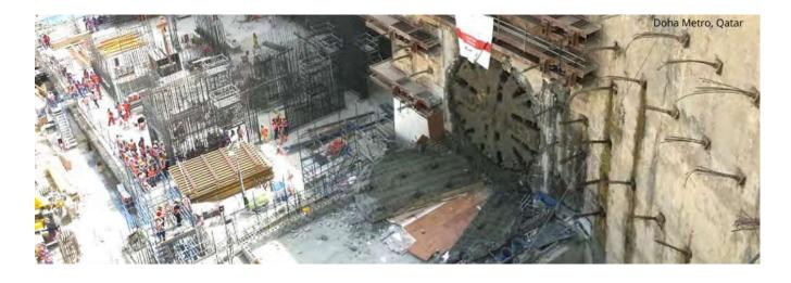
**Nordic Geo Support's ASTEC Soft Eye from Dextra** is the turnkey solution for efficient boring of reinforced concrete structures. Soft Eye facilitates the penetration of the Tunnel Boring Machines (TBM) through diaphragm walls and secant piles.
