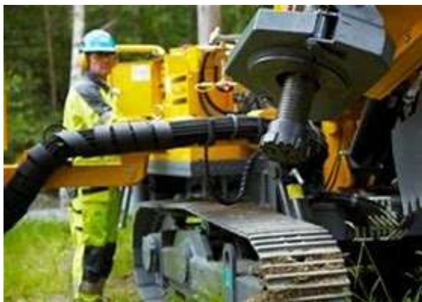
Buildings requiring integrated foundations and underpinning works
